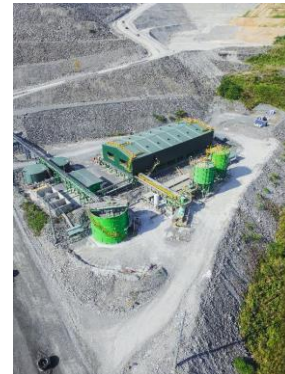
• Paste Backfill Plant
