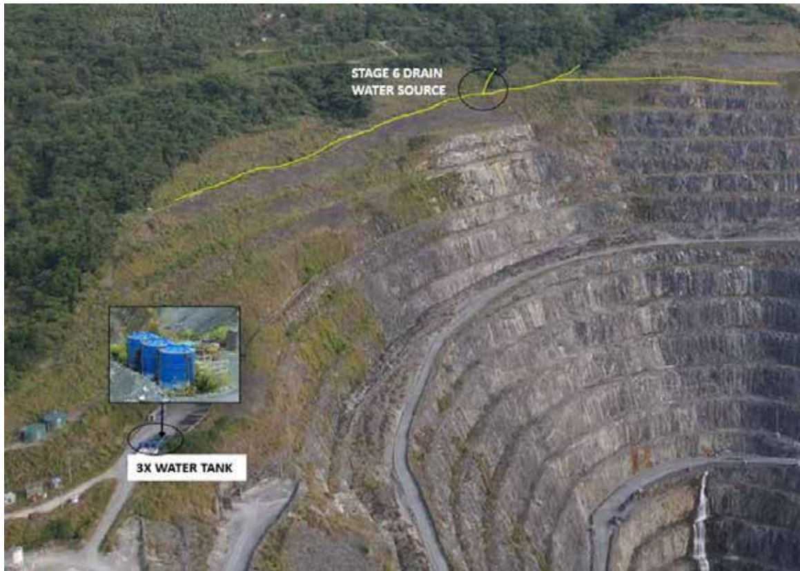
Figure 10-48. Underground Mine Water Supply
