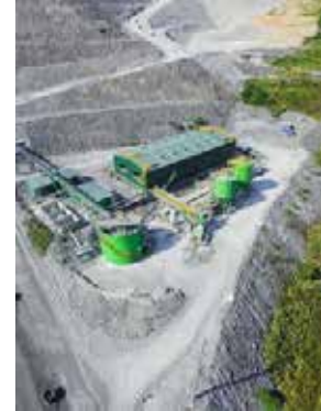
• Paste Backfill Plant
