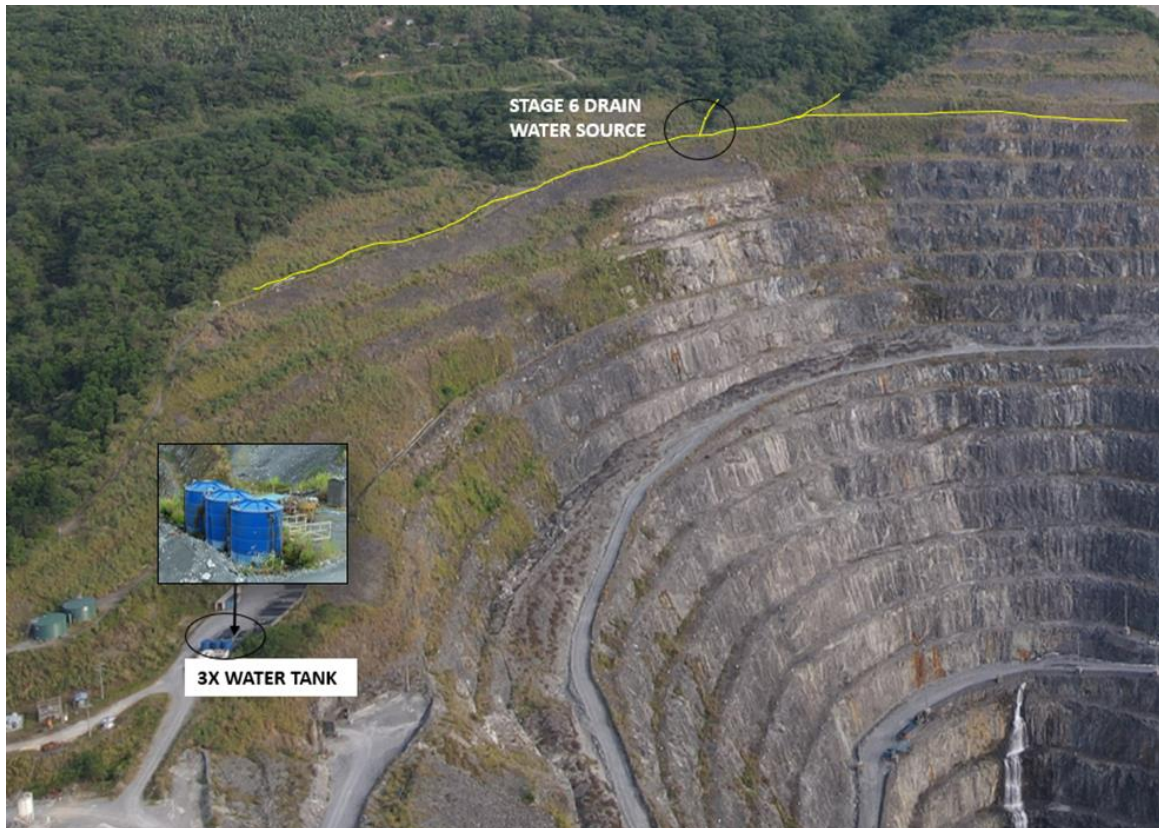
Figure 10-48. Underground Mine Water Supply
